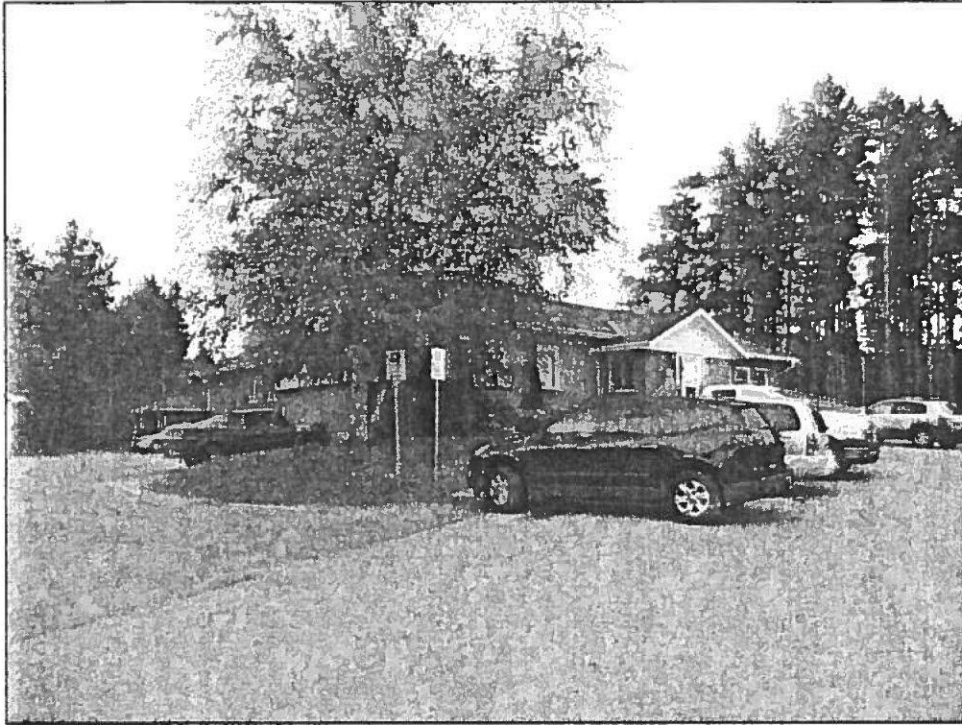
Photo 1 – Tiny Township Administration Building – South West Corner
