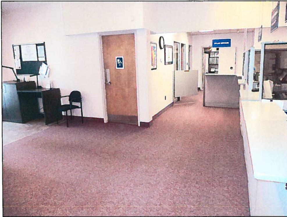
Photo 17 – The Public Washrooms are Located Too Close to the Front Counter
