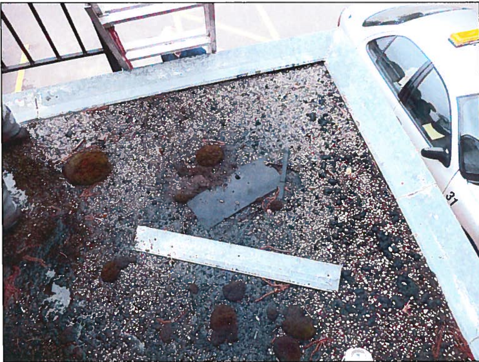
Photo 4 – Flat Roof Over Septic Inspector's Office
