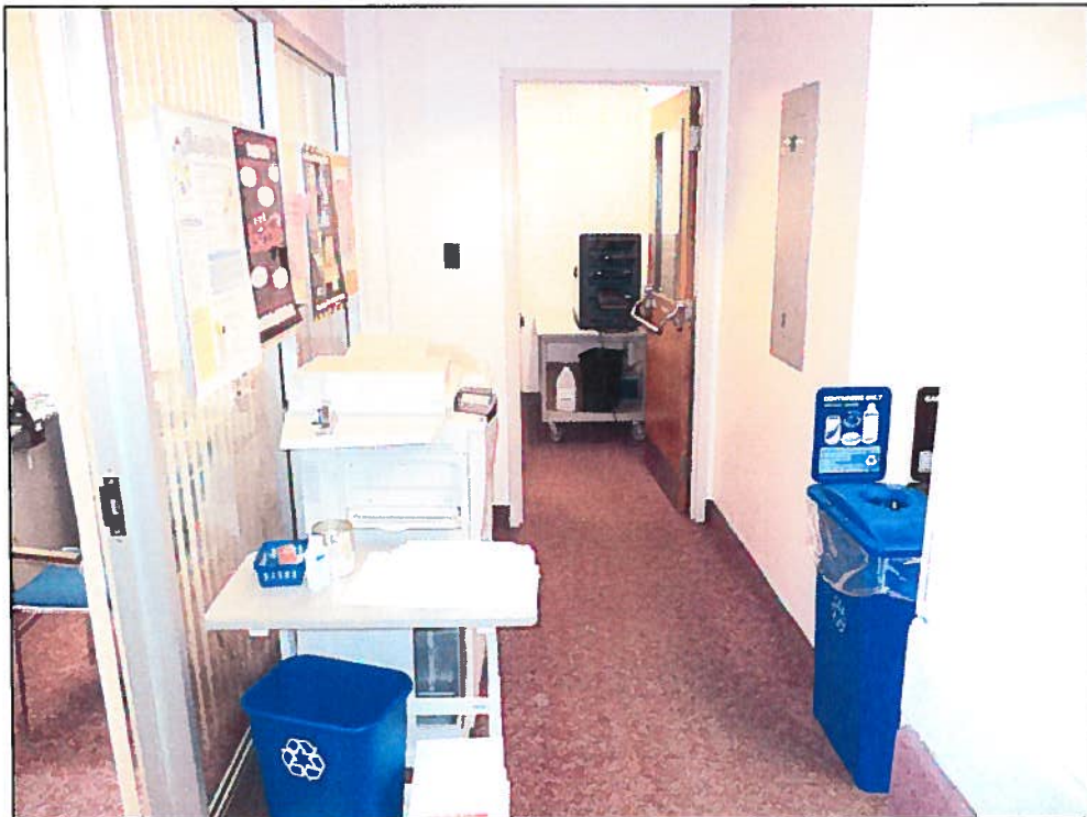
Photo 14 – The Location of Communal Printers and Correlation Services are Not Well Related to Users and Also Affects Means of Egress
