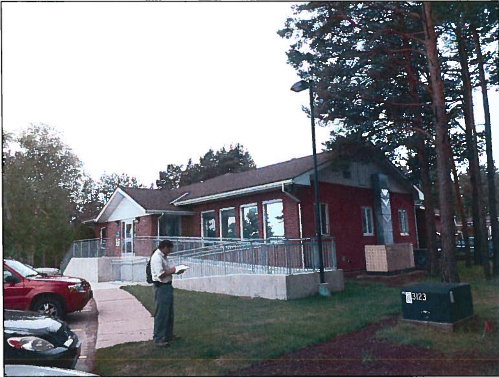
Photo 3 – Tiny Township Administration Building – South East Corner
