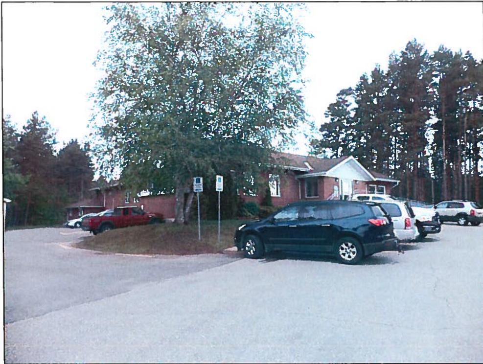
Photo 1 – Tiny Township Administration Building – South West Corner
