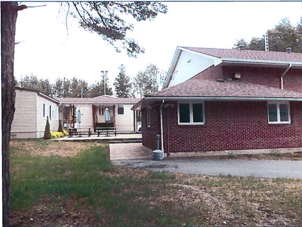
Photo 2 – Two Temporary Portable Structures at Rear of Addition
