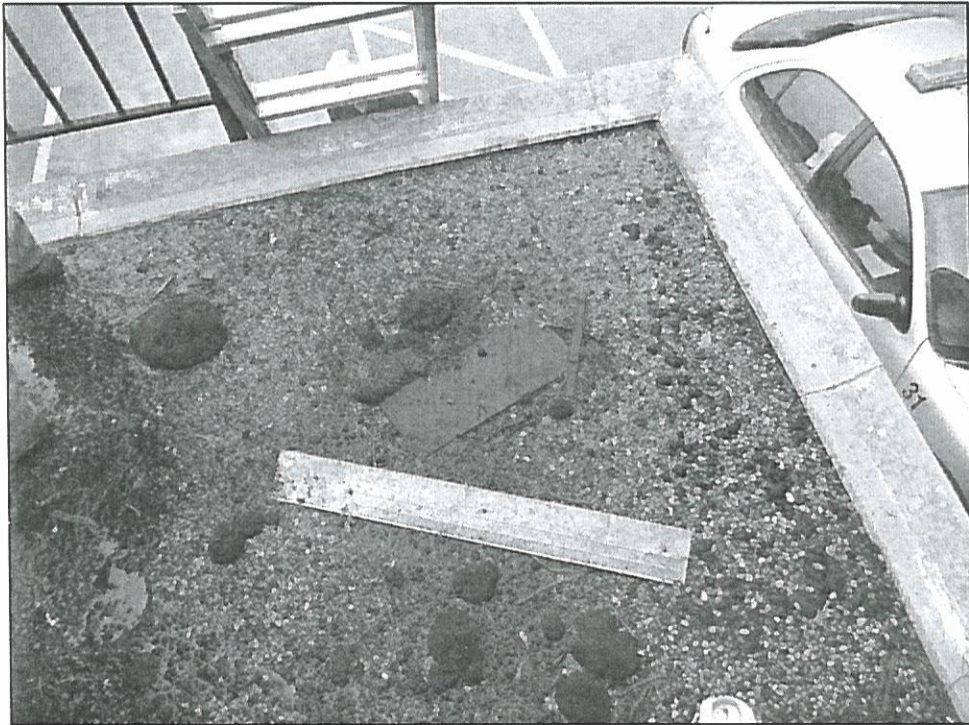
Photo 4 – Flat Roof Over Septic Inspector's Office
