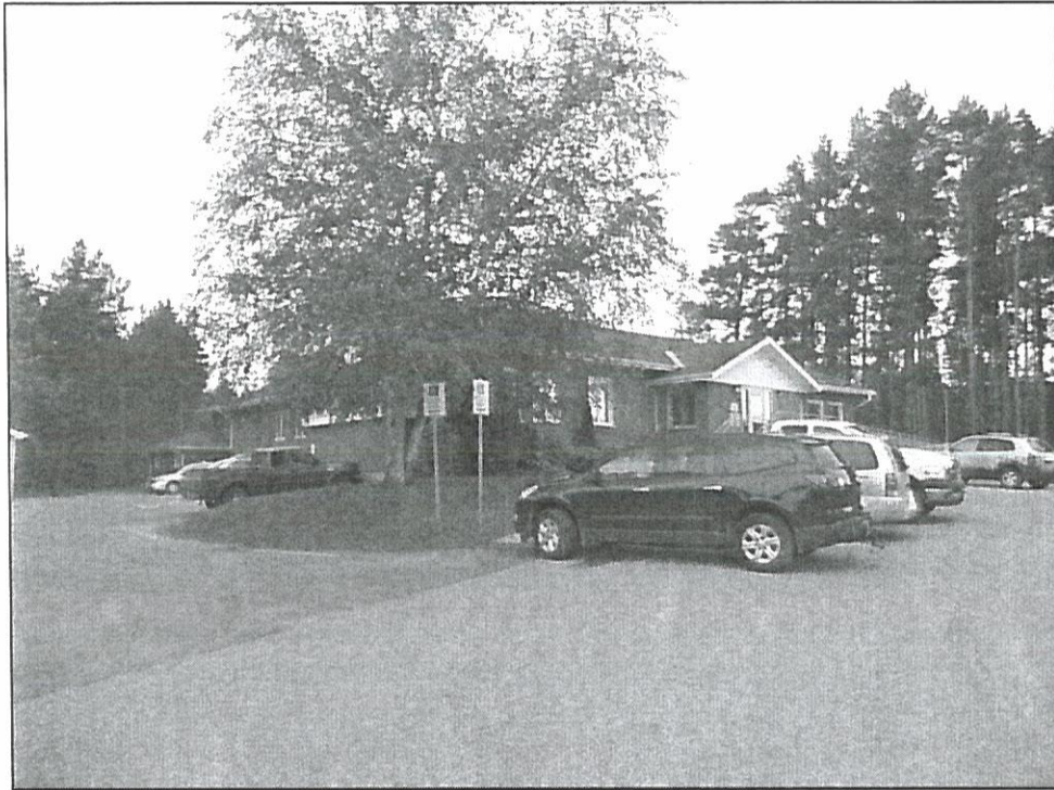
Photo 1 – Tiny Township Administration Building – South West Corner
