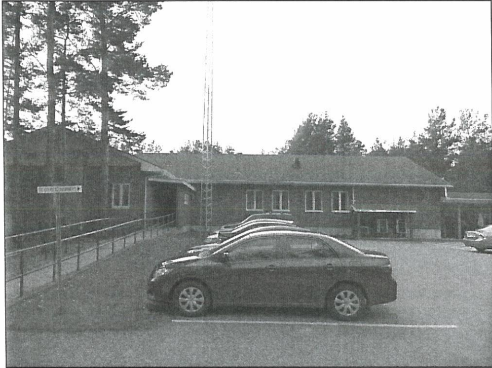
Photo 11 – Brick Paved Ramp at South Side of Building
