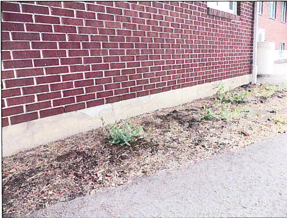
Photo 9 – Cracking at Top Course Head Joints of Concrete Block Foundation, Entrance Lobby at Northeast Corner of Addition
