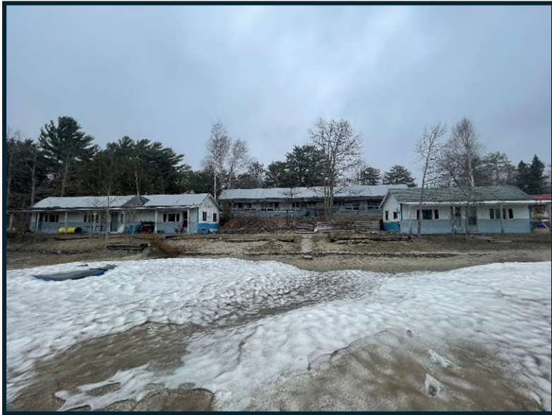
Photo 1: Taken from the beach front, towards the east showing all 3 existing structures to be demolished.
